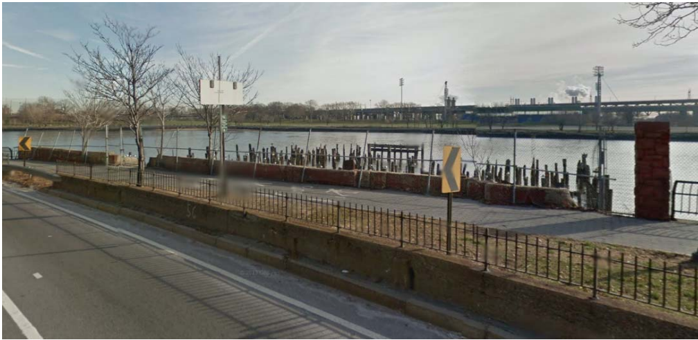
View from FDR Drive Northbound, pre-collapse
