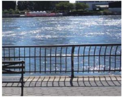
Refurbished Sea Rail
